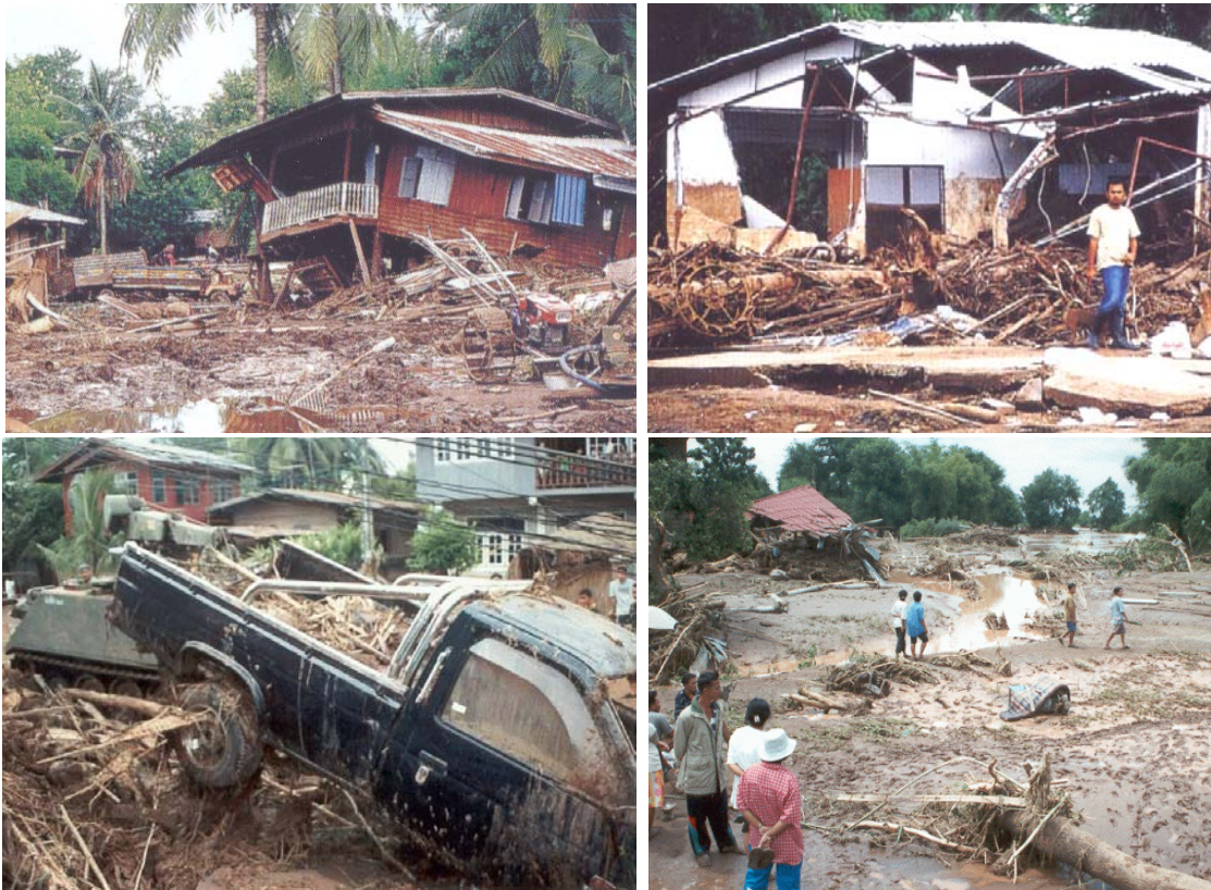
Figure 6-6 Four photographs showing some examples of seriously structural damage of houses and other infrastructures in Ban Nam Ko Yai (in the area between A and B in Figure 6-5) battered and caused by the fast-moving 8/11 flow-flood.
